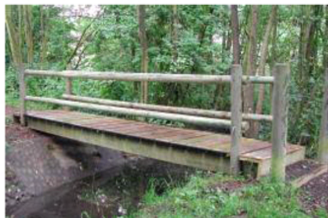
Bridge built by students from Tamworth and Lichfield College
